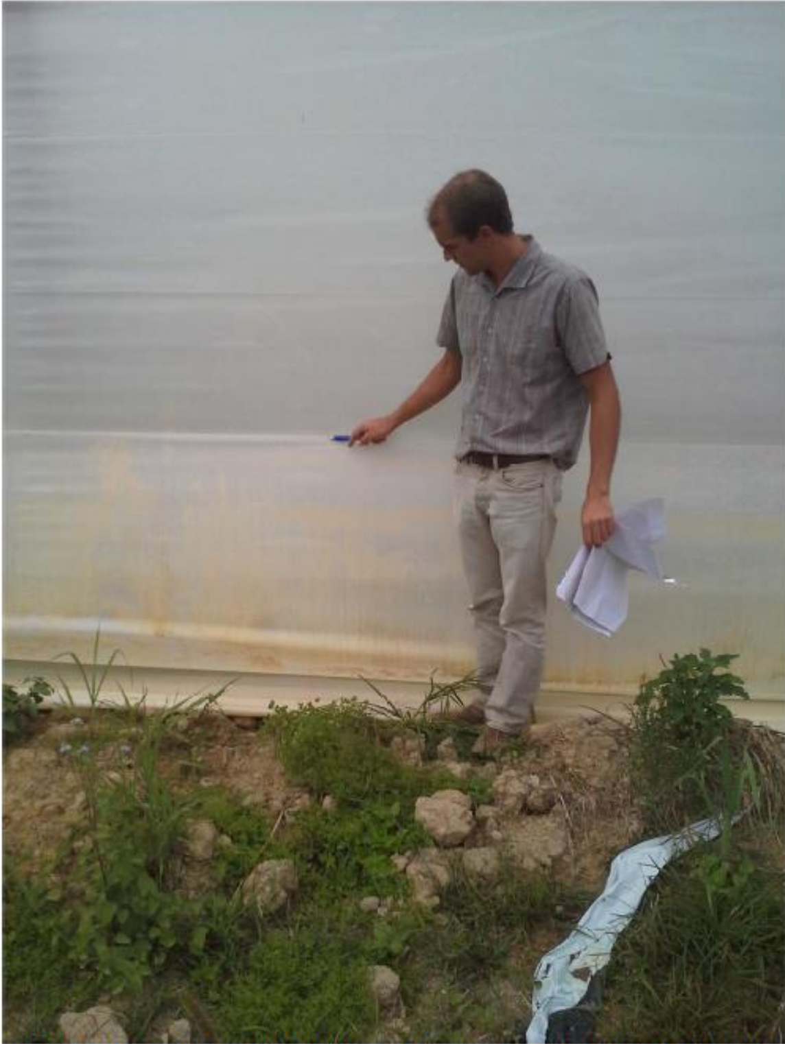
Figure.12 Markings on the north eastern corner of the shed showing the height of flood waters which went through the shed.
